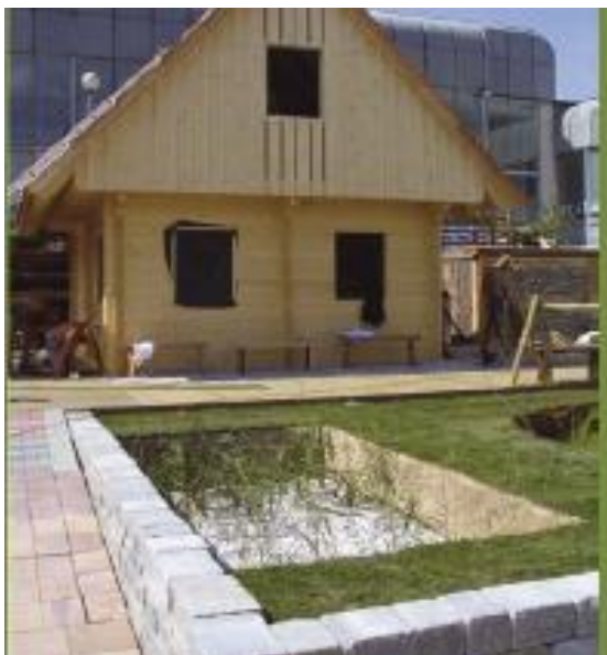
Picture 1. Constructed wetland as a water treatment facility (Limnos arhiv, 2009).
