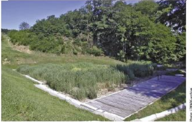
Constructed wetland for treatment of landfill leachate from a dump at Ljutomer, Slovenia
